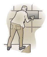
6. Brick up and seal the work hole.
