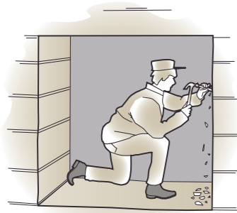
1. Hack out a work hole that is sufficiently large to insert the bottom cone just above the connector pipe.
